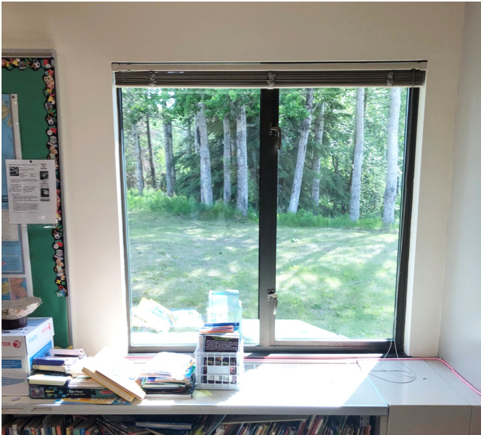
The existing windows have been partially replaced with newer, more energy efficient insulated units. The remainder will be replaced over the next few years.
