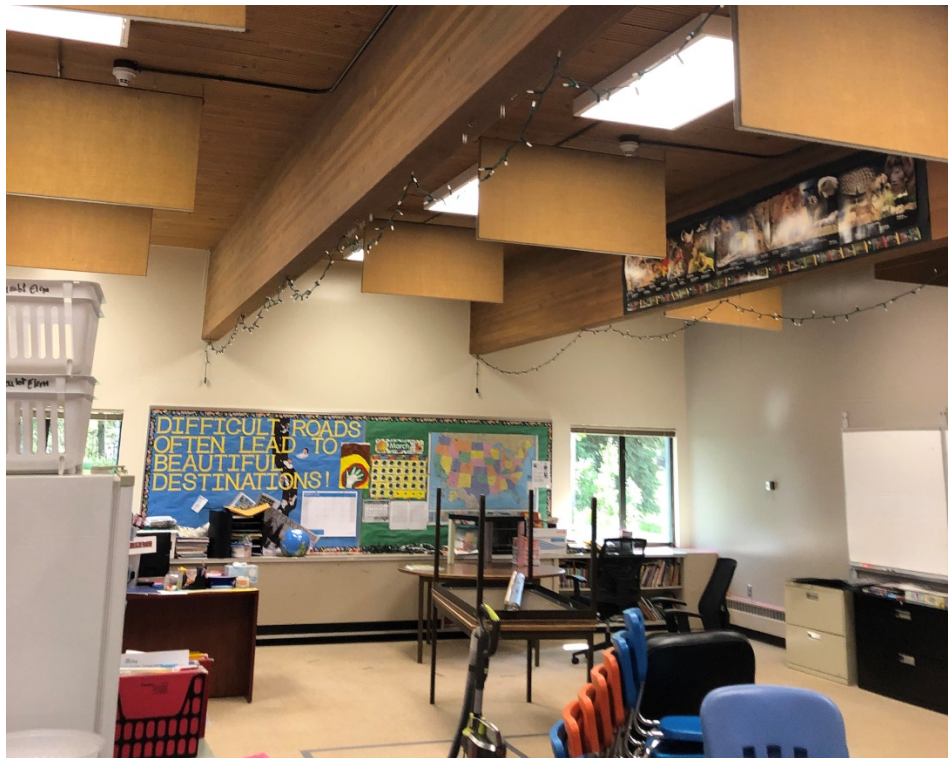
Classrooms are open to the glu-lam structure above.
