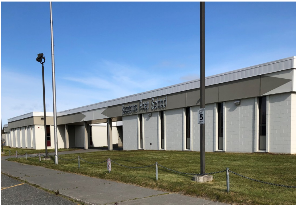
Main entry to Soldotna Middle School at the south elevation.
