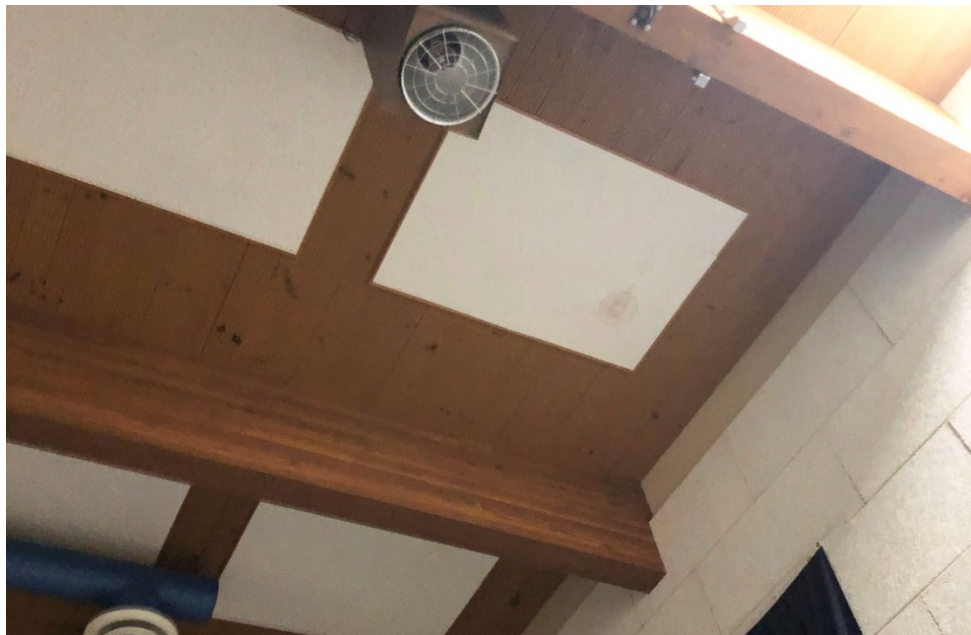
The multi-purpose space has exposed wood beams and roof decking.
