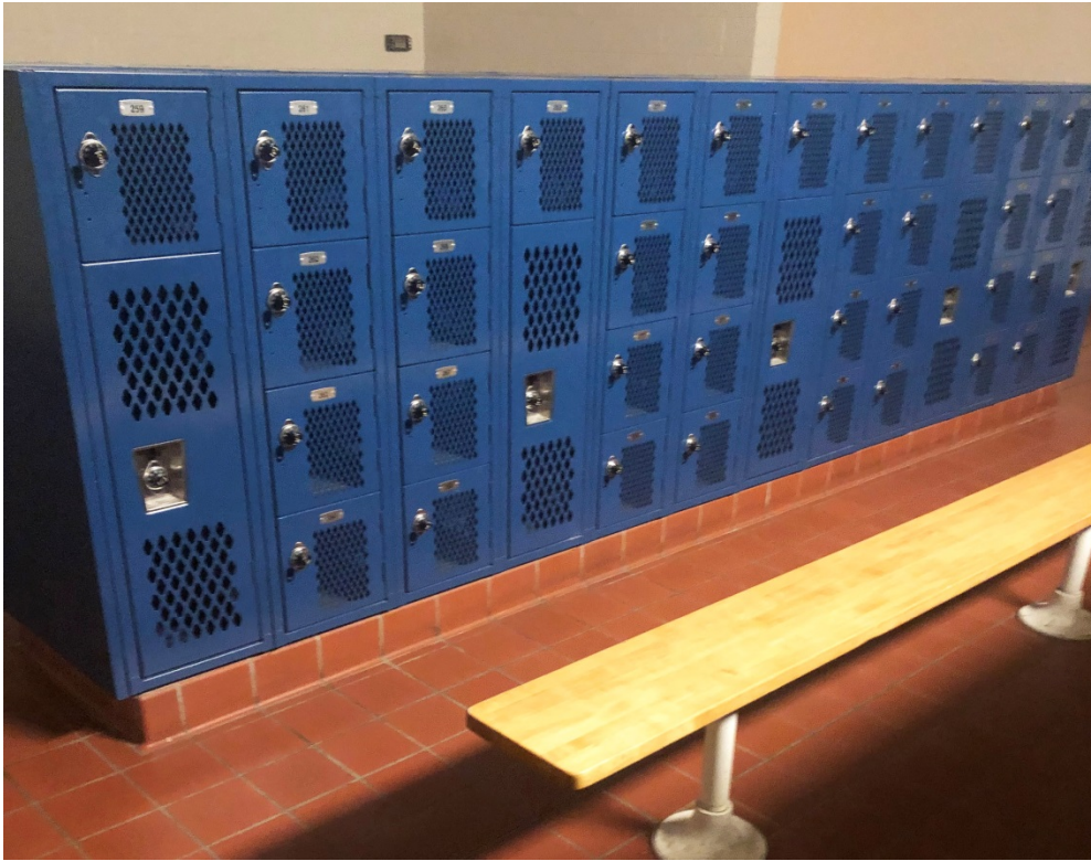
The locker rooms and shower areas are in good condition, but unlikely to be used by elementary students.
