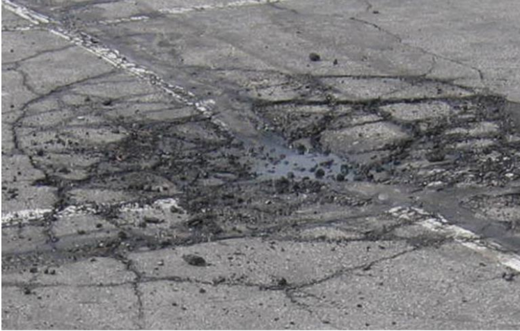
Alligator Cracking
