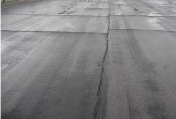
Linear Cracks
